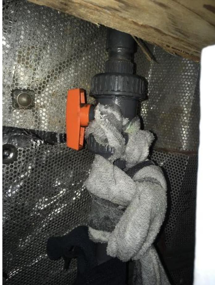
**Figure 5.** Depiction of the leaking PVC ball valve that joins pipes leading from the Jacuzzi/sea water pump to the underway system in the forward lab. The leak was tied off using rags for the duration of the mission. *Figure contributed by Lindsay Beazley.*
